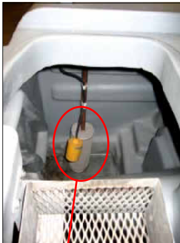
Extended Scrub (Float) Switch S7
