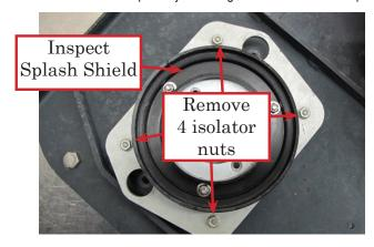
5. Flip the scrub head upright and remove each of the isolators from the brush head by removing the attaching nuts.
